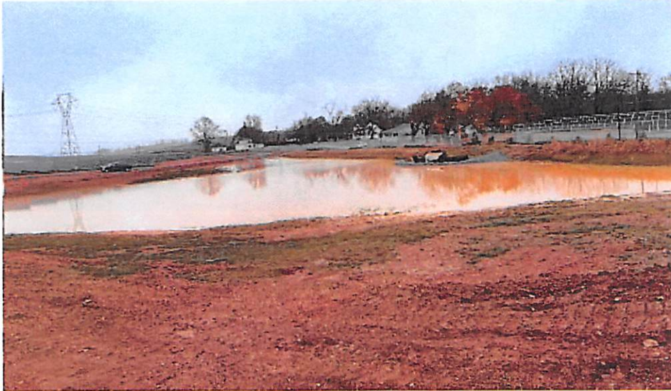
Figure 7 – Retained water in Pond 14
