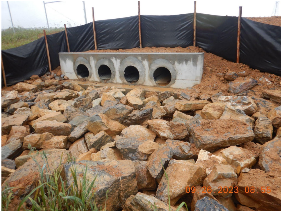
Outlet drainage area of Sediment Basin 14, discharging onto Kabletown Road
