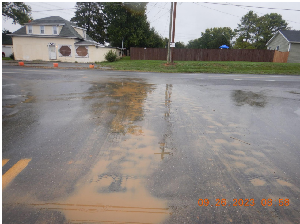
Sediment laden water laying in the road at the intersection of 115 and Kabletown Road.
