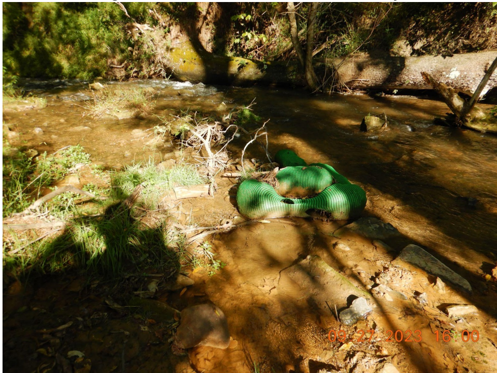
Conditions not allowable deposits into Evitts Run (39° 15' 17.2288" X -77° 49' 26.9350") from Basin 5. Filter Sock laying in creek.
