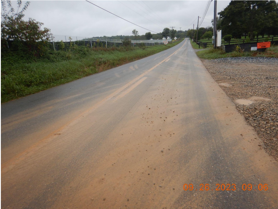
Track out from the site on Kabletown Road.
