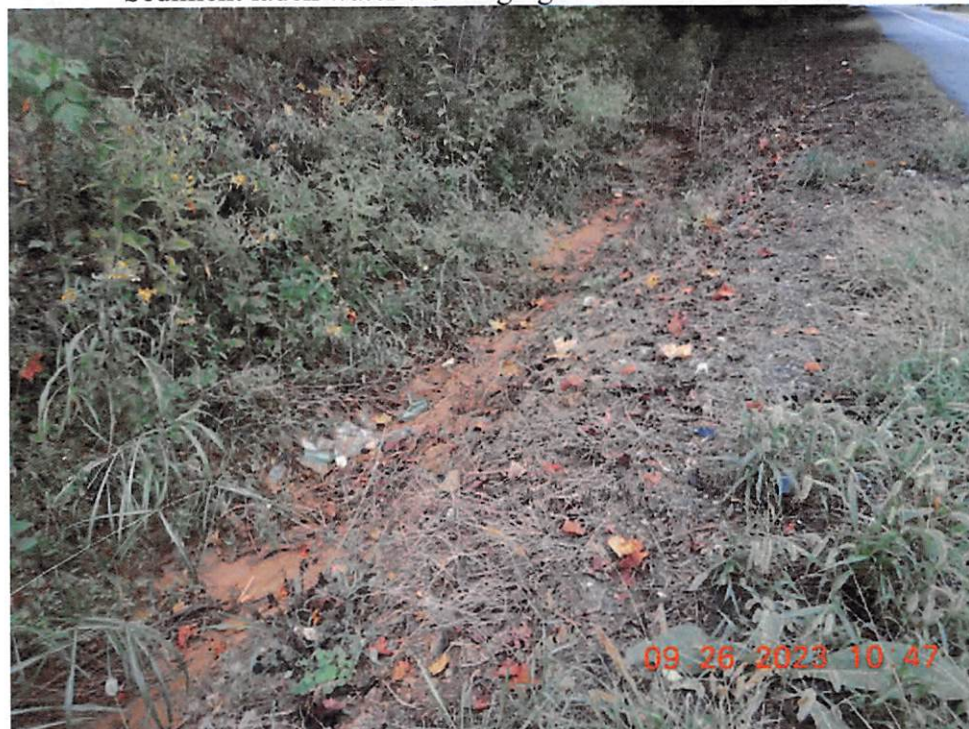
Sediment laden water from Sediment Basin 6 entering into an ephemeral UNT of Evitts Run (39° 15' 33.3189" X -77° 49' 30.6042").
