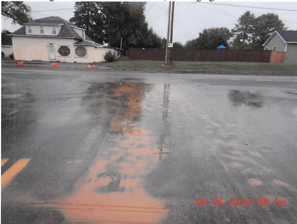
Sediment laden water in the road at the intersection of 115 and Kabletown Road.
