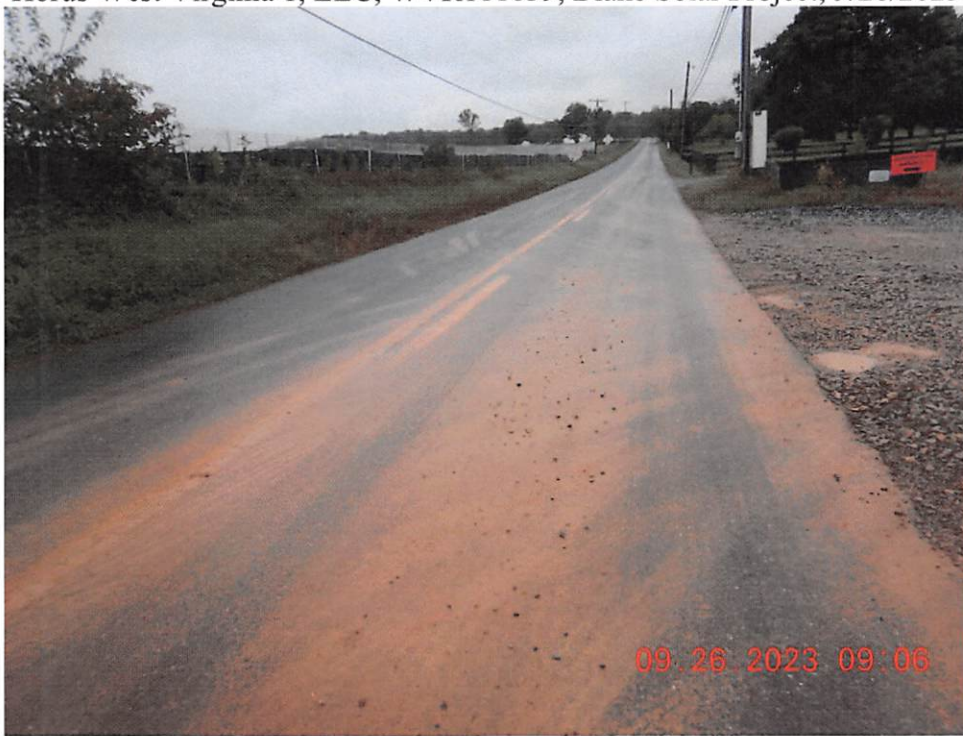
Track-out from the site on Kabletown Road.
