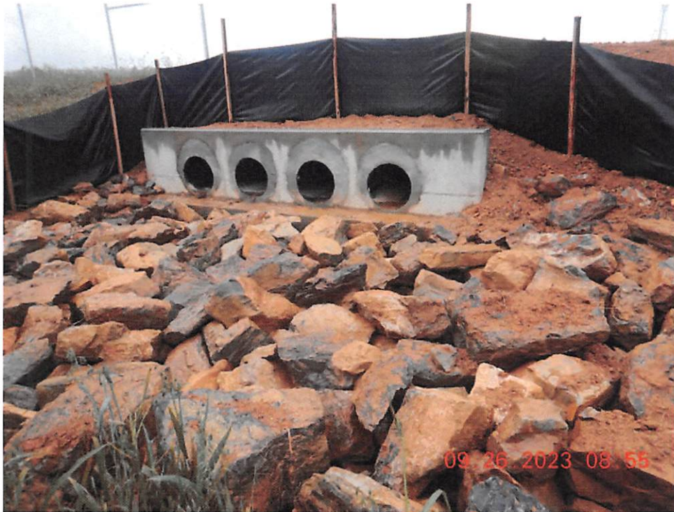
Outlet drainage area of Sediment Basin 14, discharging onto Kabletown Road
