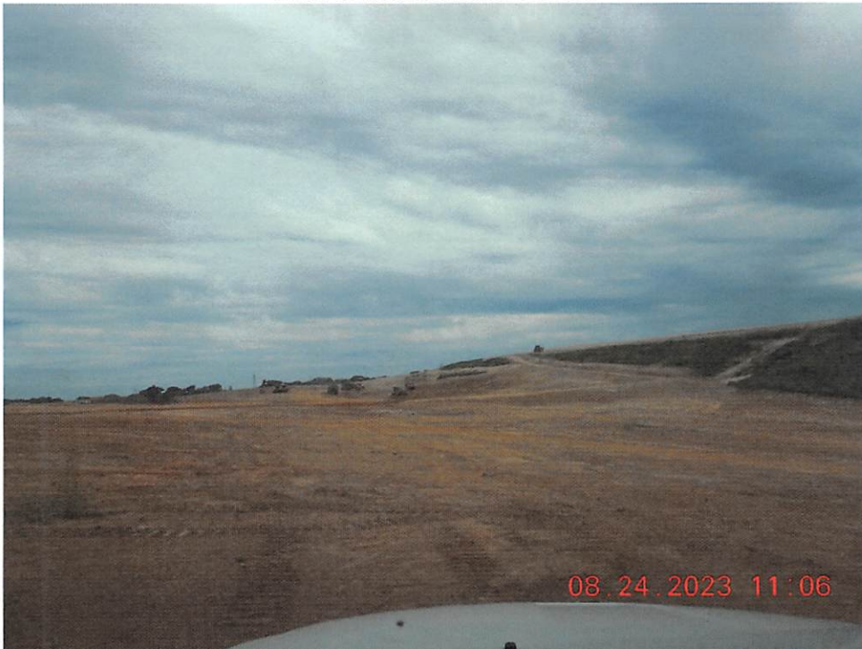
Area that lacks stabilization.
