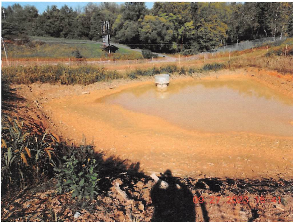
Sediment Basin 6 with accumulated deposits.
