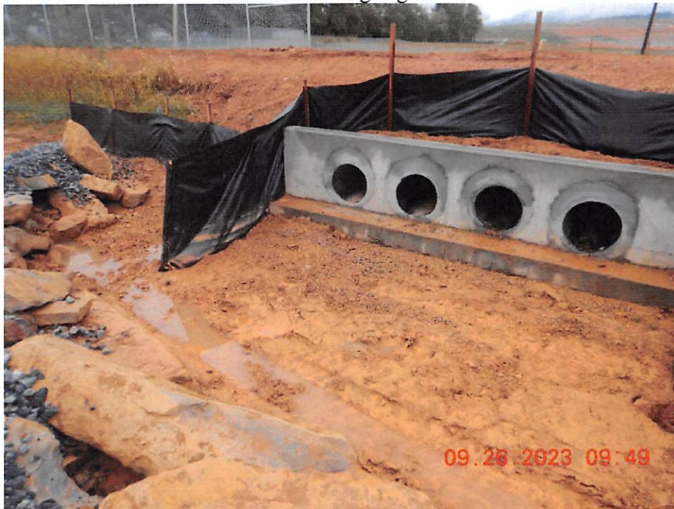
Outlet for stormwater pond 14 has been installed. Sediment laden water leaving site through outlet.
