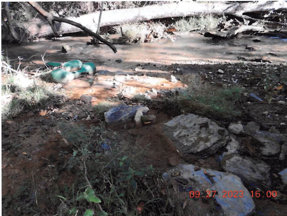
Conditions not allowable - deposits in Evitts Run (39° 15' 17.2288" X -77° 49' 26.9350") from Sediment Basin 5.
