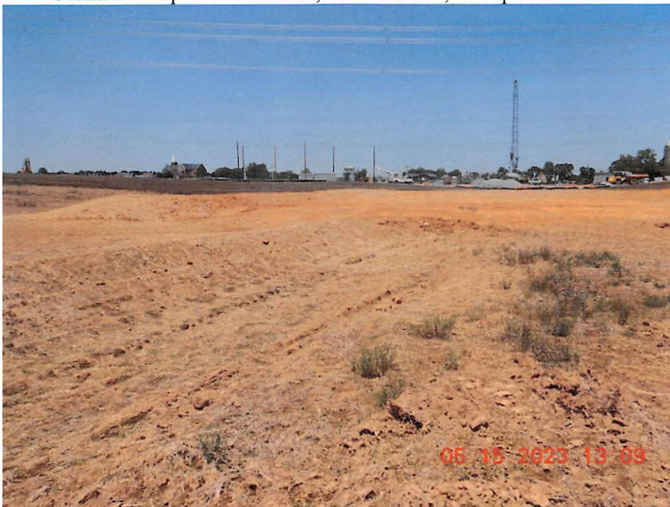
Clean water diversion is not vegetated prior to being put into use.
